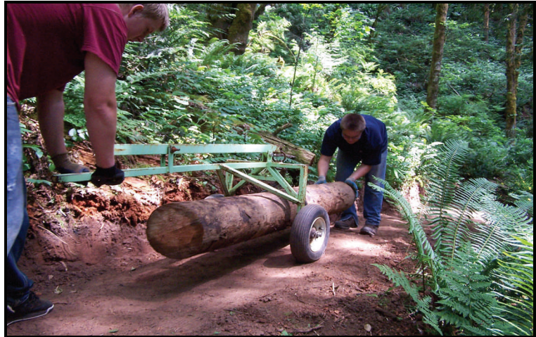
Two of the Community Solutions summer crew use a junior arch to move a large pole into place for a stream crossing on Little Buckner Trail.
