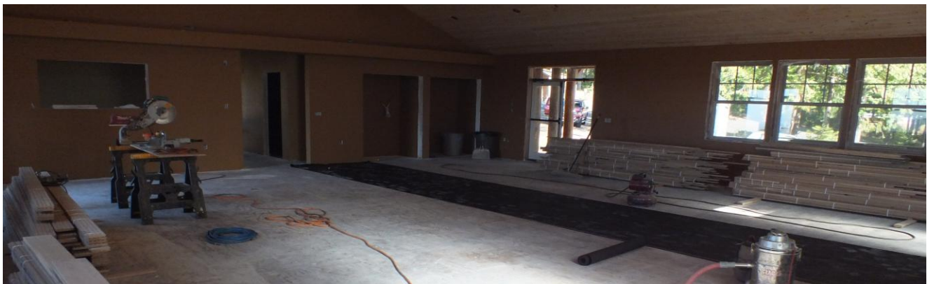
Forest Hall flooring and installation.
