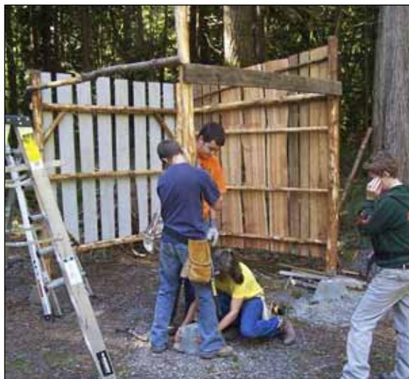
**Youth crew members used primarily native materials found at Hopkins to build two rain shelters now found in our woodland. The shelters are built from small Douglas-fir poles as structural members, assembled with mortis and tenon joints; and cedar shake cut by hand for roof and siding.**
