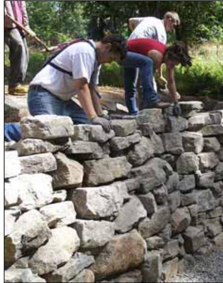
**The Clackamas County Youth Corps crew was given 35 tons of rock and a simple picture of how to stack a dry wall, and built the wall like a puzzle—sometimes pulling rock out to fit another into place.**
