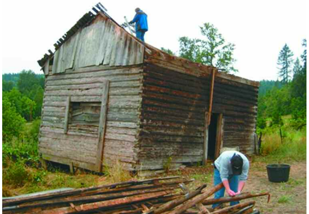
Volunteers working on the dismantling of the Molalla Log House.
