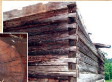
small functional building with a compact and efficient design. It measures 18’ x 25’ and has a gable roof. Large mudsills rest on foundation rocks and support 17 additional horizontal logs on each side to make the 1½ story building. The ground floor appears to have been a single room and the second floor loft provided a very usable space with standing room in the middle.
